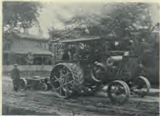
Fig. 8.—Scarifier operated by Traction Engine.
